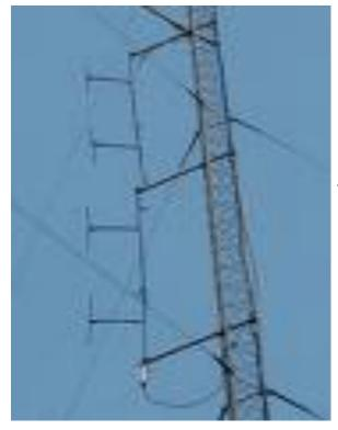
Z<sub>o</sub>= 276 log 2(S/D) S=Distance between and D=diameter
